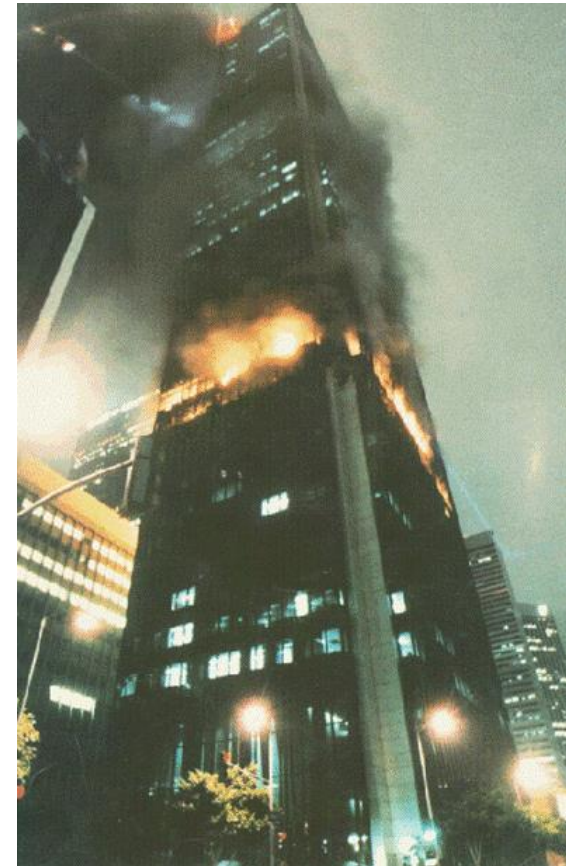
1st Interstate Bank, Los Angeles, CA.
