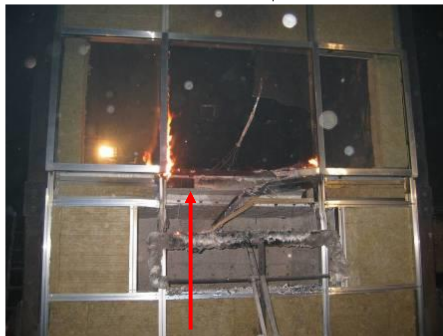
Less than 20 minutes of exposure melts aluminum transom.
